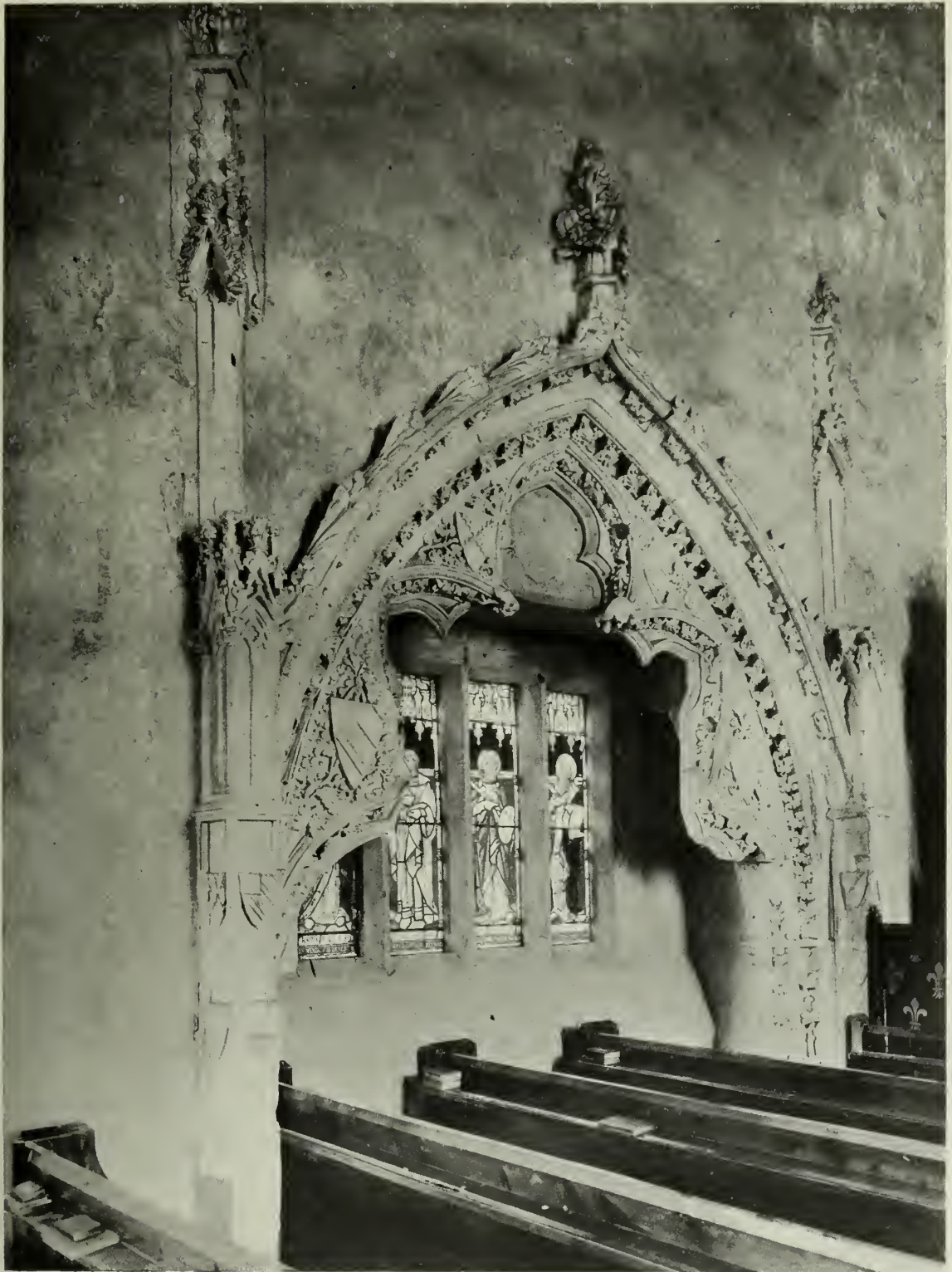
BELCHAMP WALTER: PARISH CHURCH OF ST. MARY THE VIRGIN. Chantry recess on N. side of Nave; c. 1325.
